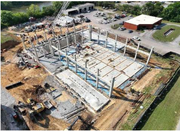
Aerial View from Northeast
