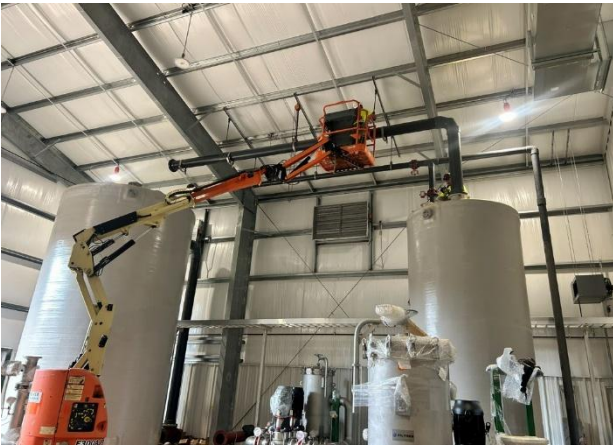
Piping installation in Chemical Building
