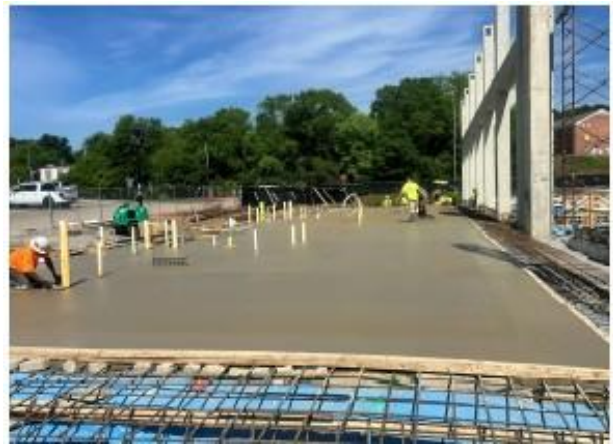
Administration Slab Placed
