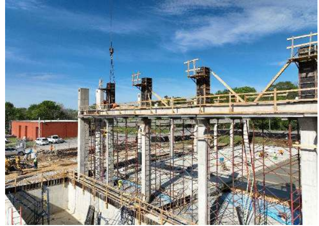
CMF Bridge Crane Supports
