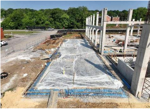
Preparing to place Administration Slab
