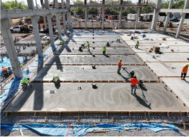
Eastern RO Floor Placed
