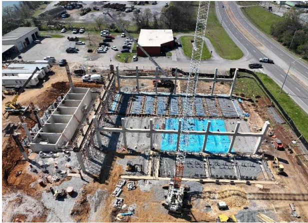
Aerial View from Northeast
