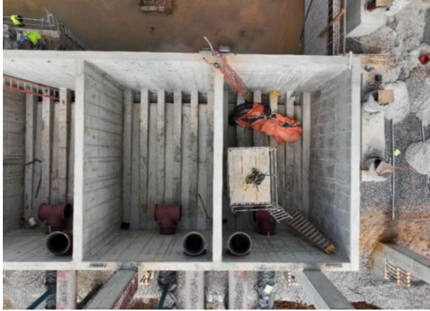
CMF Basin Piping Installation
