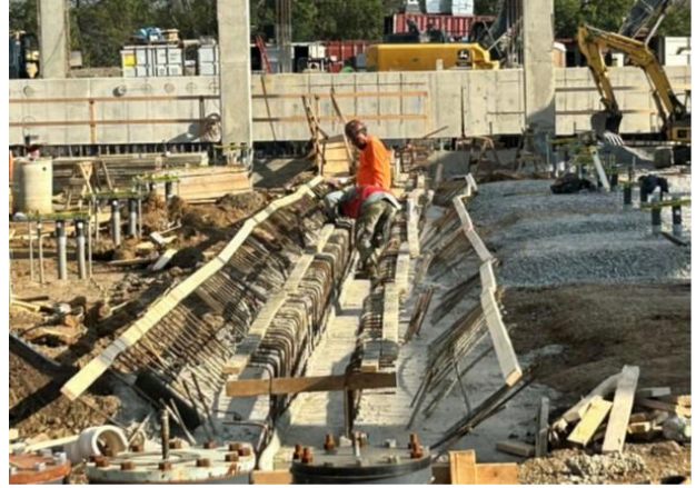
Trench Drain Forming and Pouring
