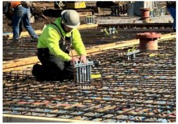
Installing RO Unit Ground Wiring
