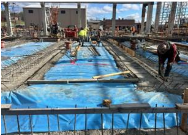
Preparing to Place Floor
