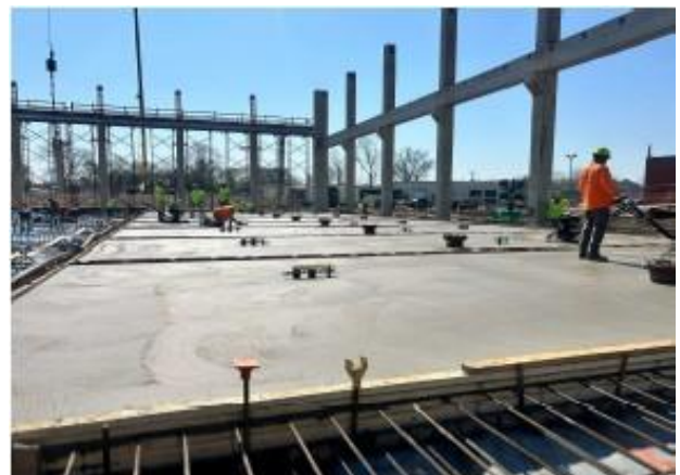
Western RO Floor Placed
