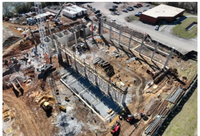
Aerial View of Main Process Building
