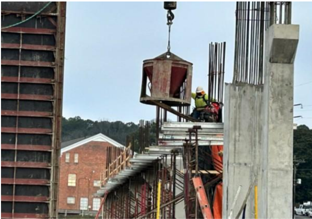
Pouring Bridge Crane Elevated Support Beam
