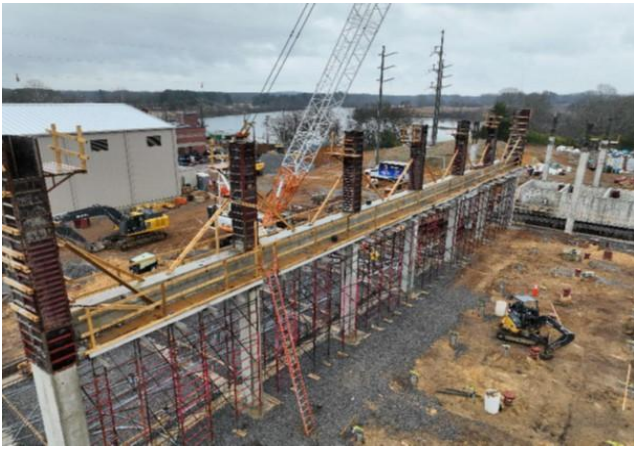
Column extension above Bridge Crane Beam
