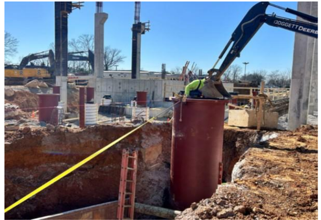
Underground piping installation
