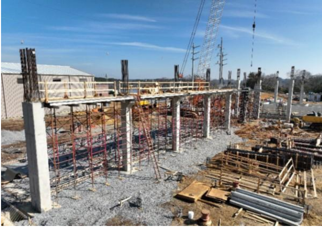
Forming Bridge Crane Elevated Support Beam
