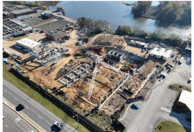
Aerial View from Northwest
