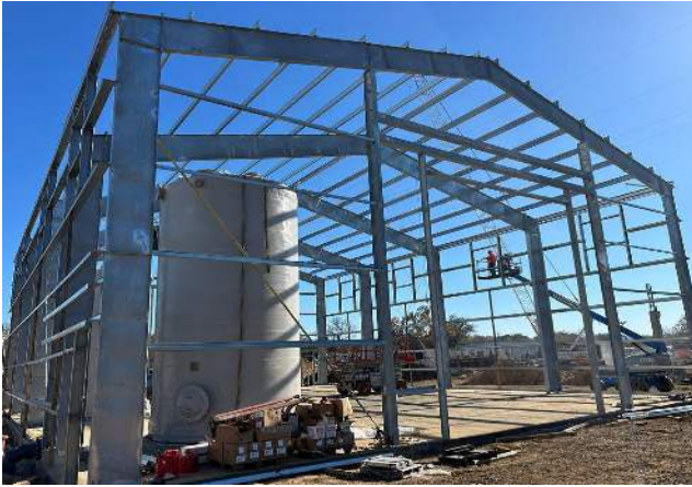
Chemical Building Framework
