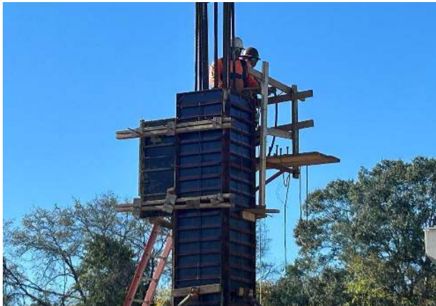
Bridge Crane Support Beam Form/Pour
