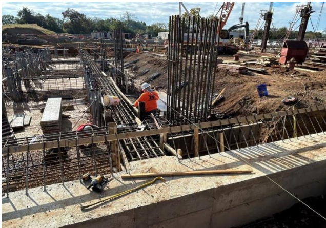
Grade Beam Form/Pour
