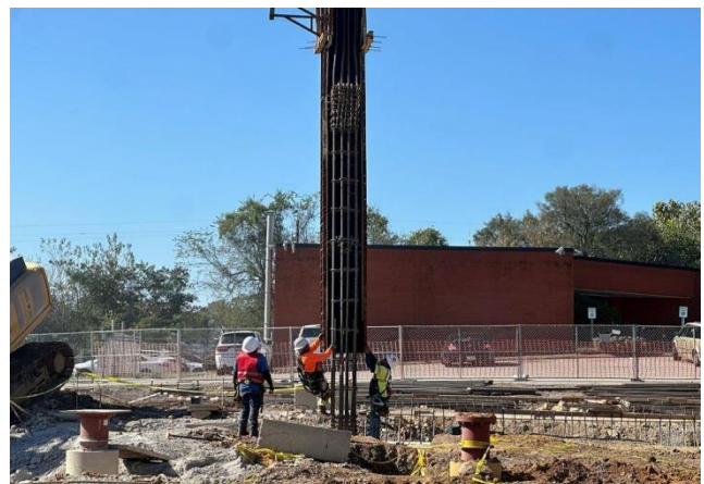
Bridge Crane Column Form
