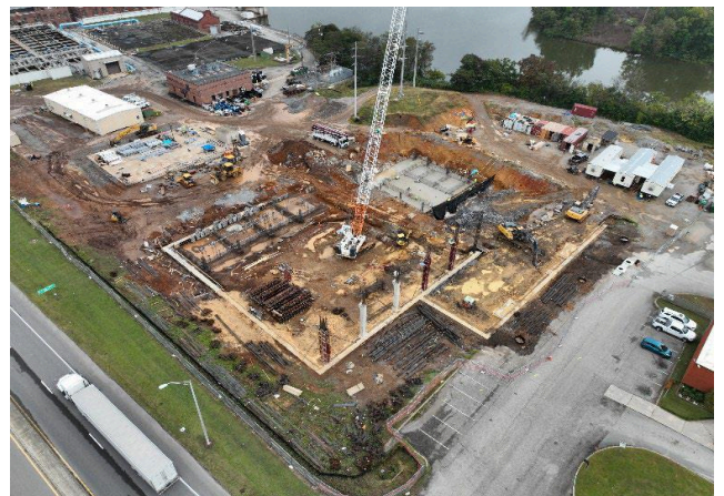
Aerial View from Northwest
