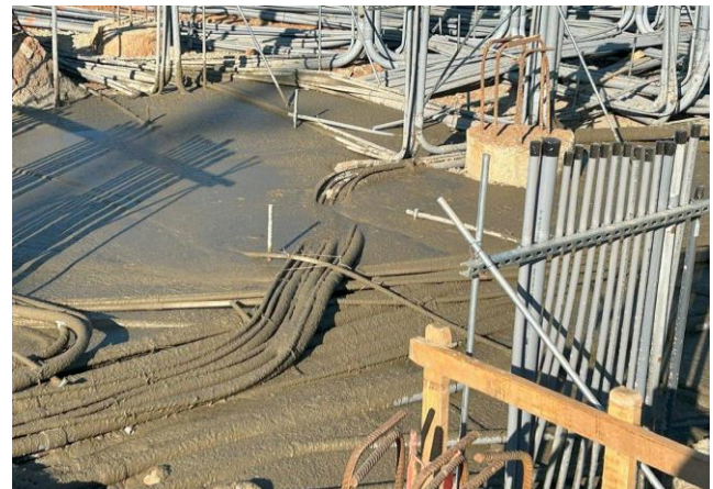
Flowable Fill in Electrical Room Floor
