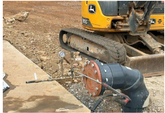
Hydrostatic Pressure Test
