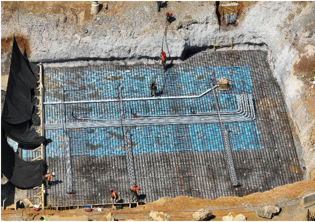
Rebar grid in the CMF Area Floor
