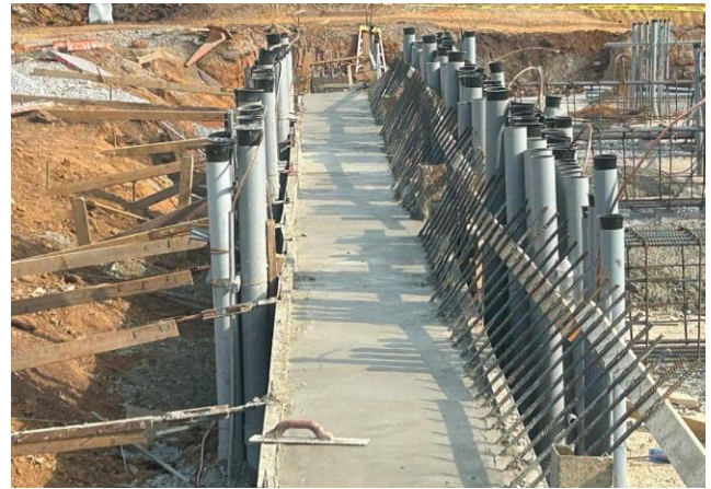
Grade Beam, with Under Slab Conduit
