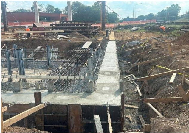
Grade Beam Form/Pour
