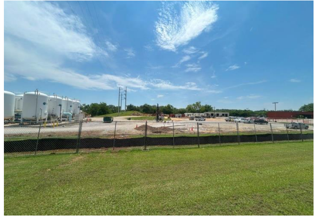
Construction Fencing Installed
