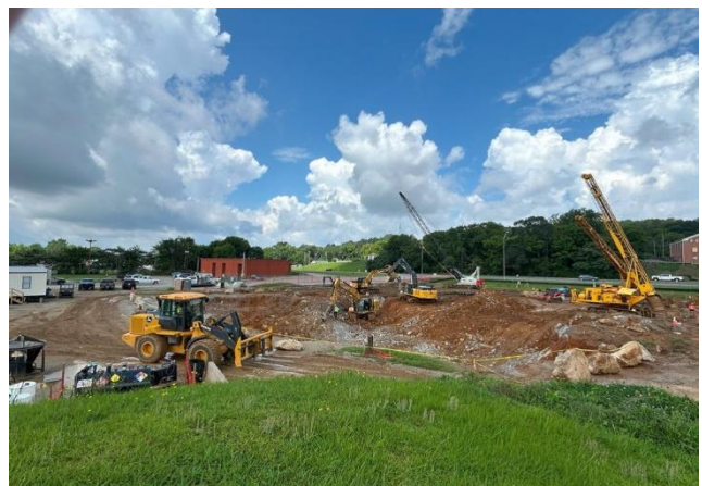
Process Building Excavation
