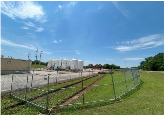
Construction Fencing Installed
