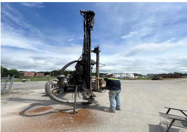
Pier Subsurface Investigation
