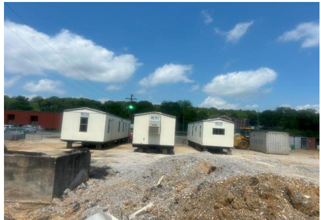
Job Trailers Arrived & Set Up
